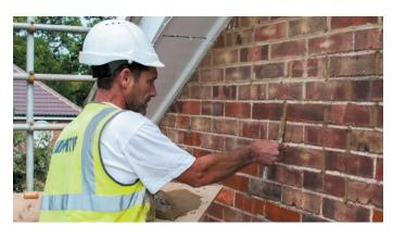
The curing time will depend to a large extent on the chosen repointing mix (e.g. mixes containing cement will cure more quickly than those based on pure lime). During the curing period mortar should be protected from frost and should be prevented from drying out too quickly. In dry, windy or warm weather it may be necessary to spray the surface of the wall occasionally or cover the wall with damp hessian to allow a proper set, particularly where a lime mortar has been used.
